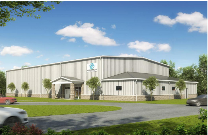
Newly-constructed Boys and Girls Club of Walker County
