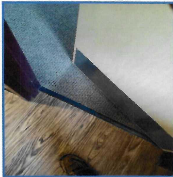
City of Huntsville / Fire Department / Transition strip from quarters to hallway. New floor covering in hallway. Quarters carpers have been cleaned.
